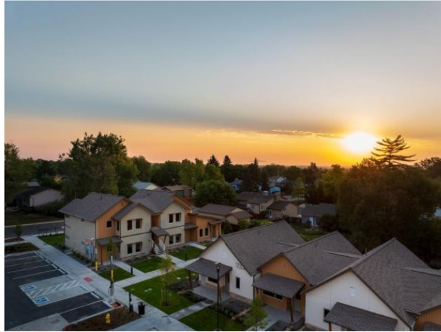
The Grove at Cottonwood in Broomfield, Colorado, provides 40 permanent affordable rental homes centered around accessibility and inclusion. (Matthew Staver)
