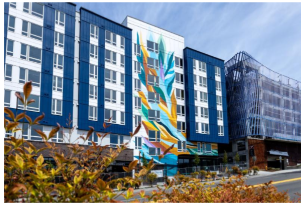
Developed by Mercy Housing Northwest, Connection Angle Lake brings new housing opportunities to people with IDD in SeaTac, Washington. (Courtesy Mercy Housing)
